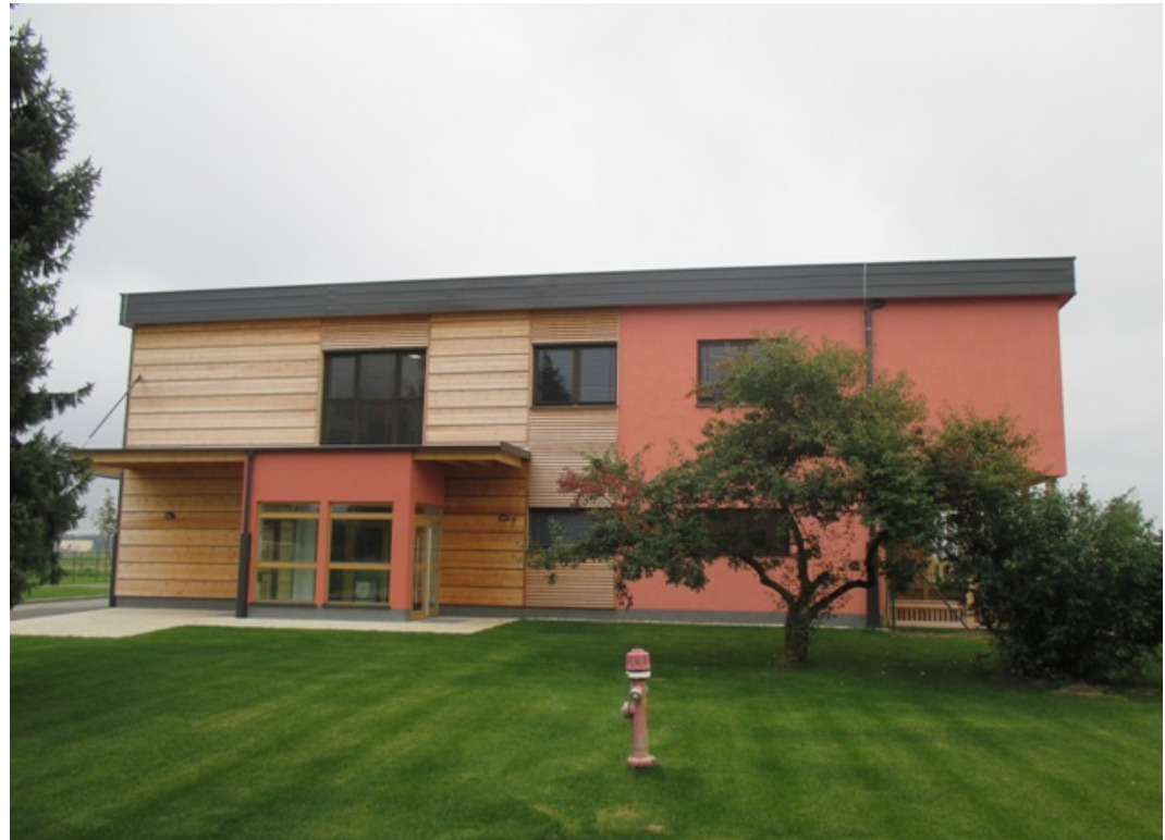
Eastern (above) and western façade © Dalibor Šošarič
